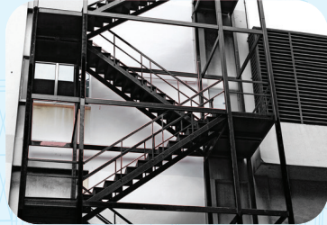
Tangga Besi / Metal Staircase
